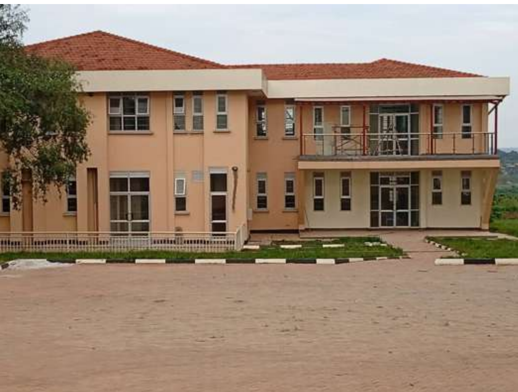
The Brand-New Office and classroom block built using ACE II funds
